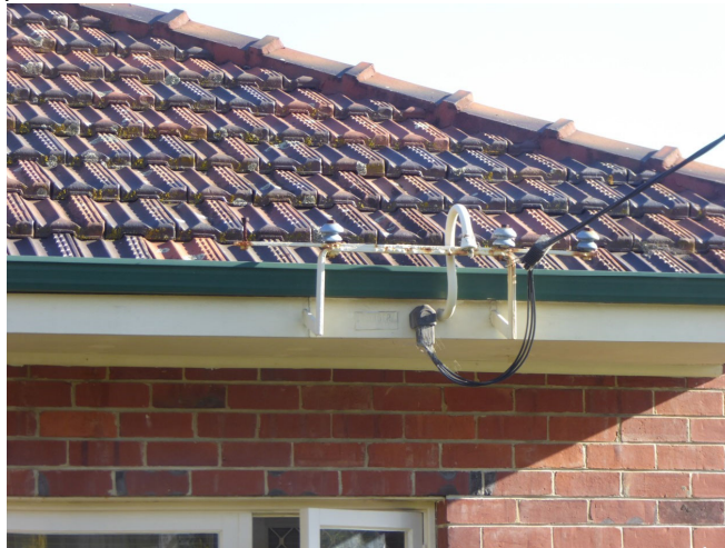
Typical roof connection bracket
