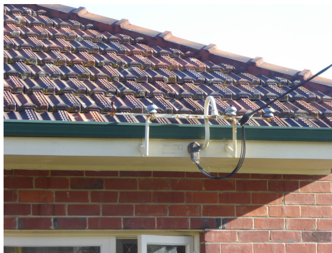
Typical roof connection bracket
