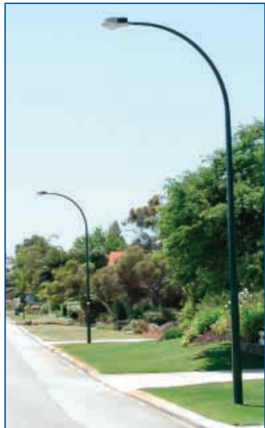
Rossmoyne Underground Power Project
